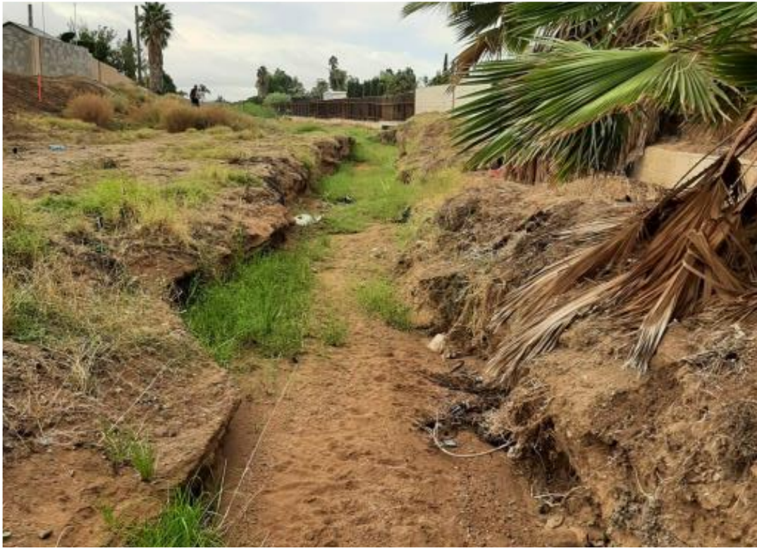
View of drainage channel looking south
