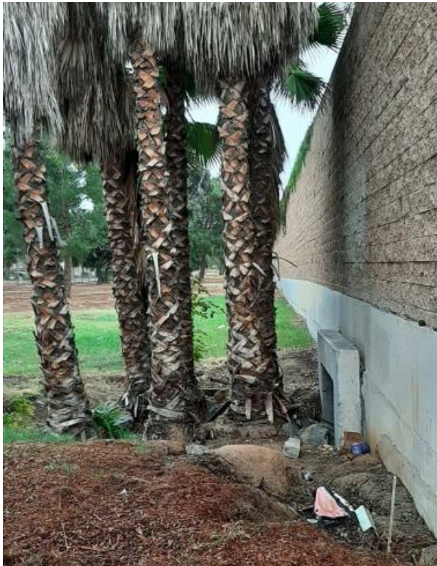
View at southern boundary looking west
