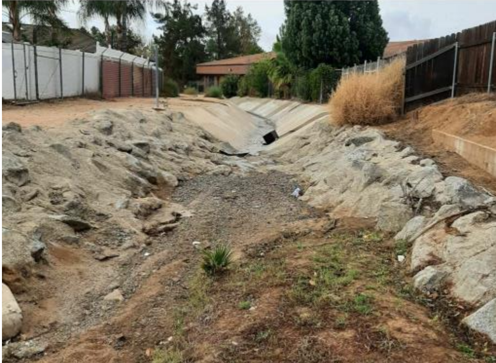
View of drainage channel looking south
