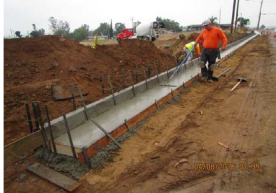
Elsworth Street and Sherman Avenue Sidewalk Improvements
