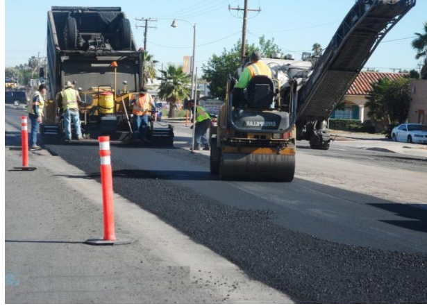
Pavement Trench Repair
