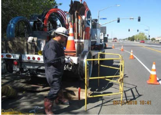
Citywide Fiber Optic Communications Expansion
