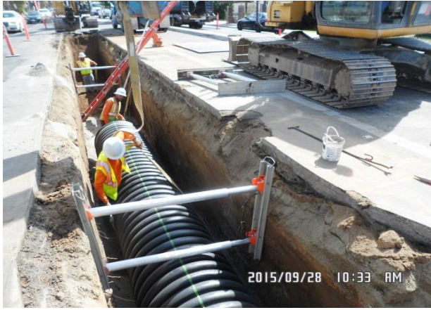
Storm Drain Trench Installation
