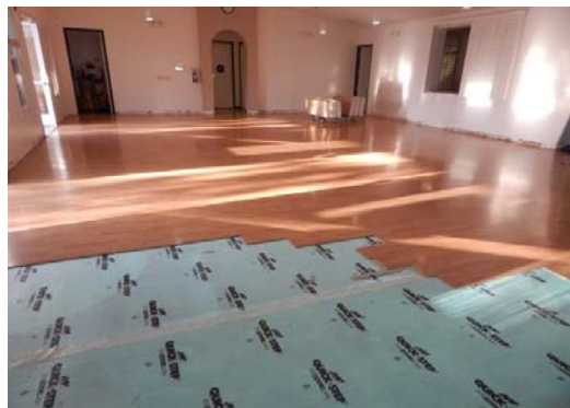
Towngate Community Center Renovation
