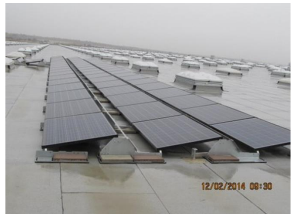
Solar system for Deckers Outdoor
