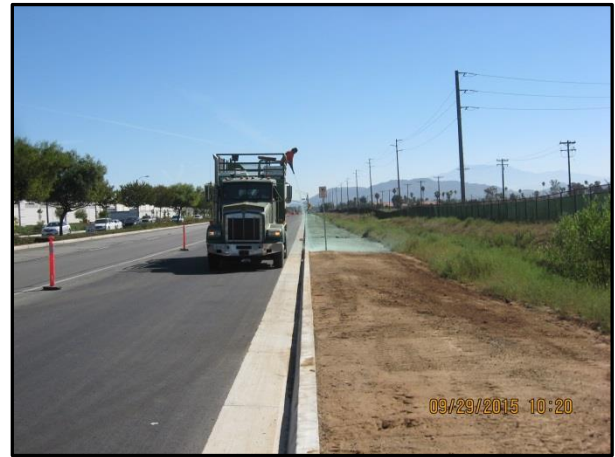
Cactus Avenue: Hydroseeding along roadside
