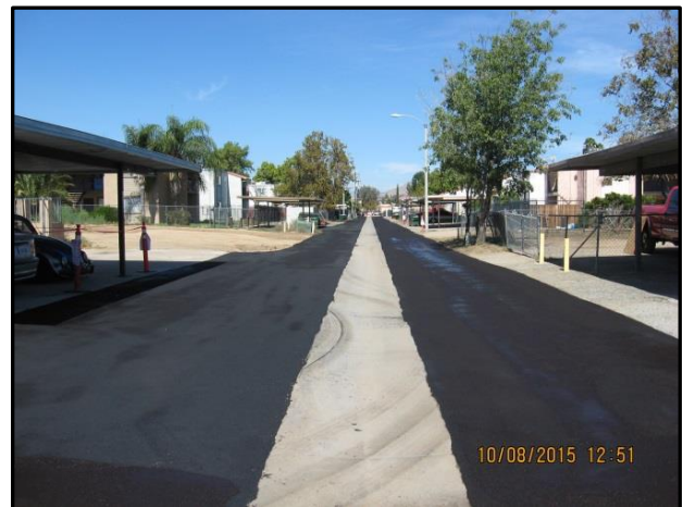
Warner Ranch Alley: After Slurry Seal
