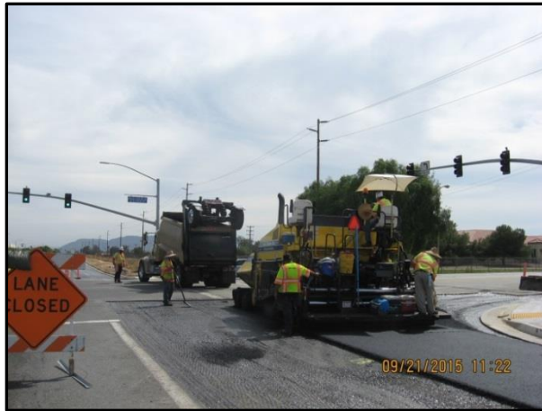
Cactus Avenue: Asphalt Cap Paving
