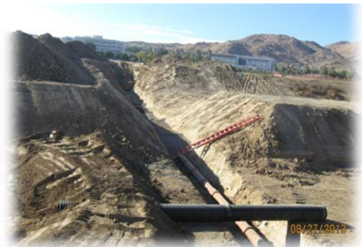
Trenching of the easterly sewer lateral.
