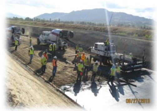
First of the Line F channel bottom concrete slabs to be poured.
