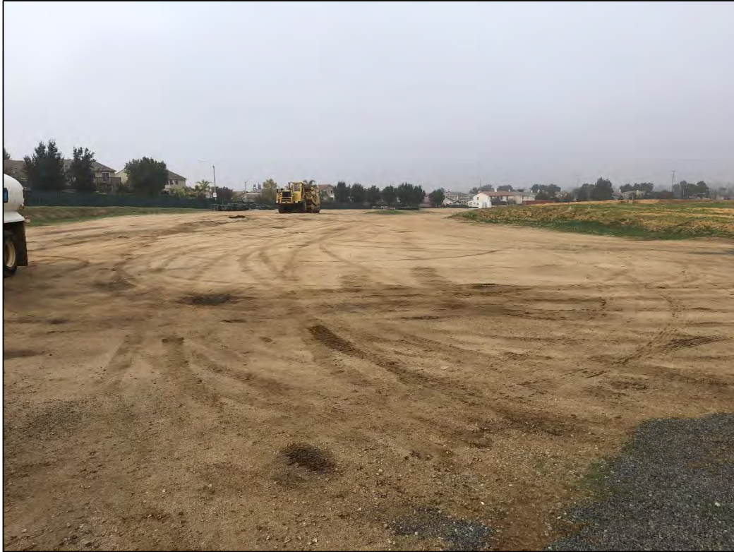
Looking north-west across the Project site.
