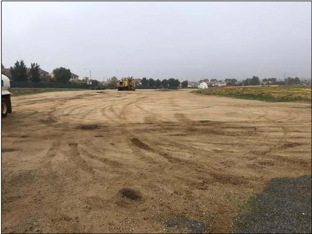
Looking north-west across the Project site.
