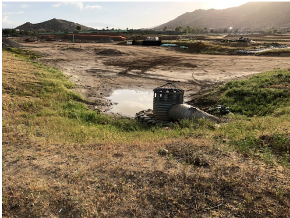
Figure 6: Overview Project Photo North East From Southwestern Corner of Project.
