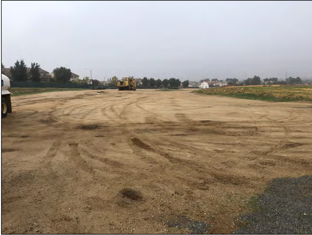
Looking north-west across the Project site.
