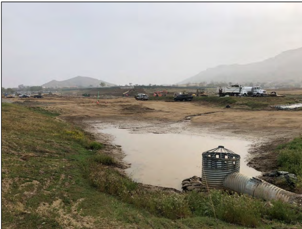
Retention Basin located on the northwestern most portion of the site to capture and retain the nuisance water and runoff.
