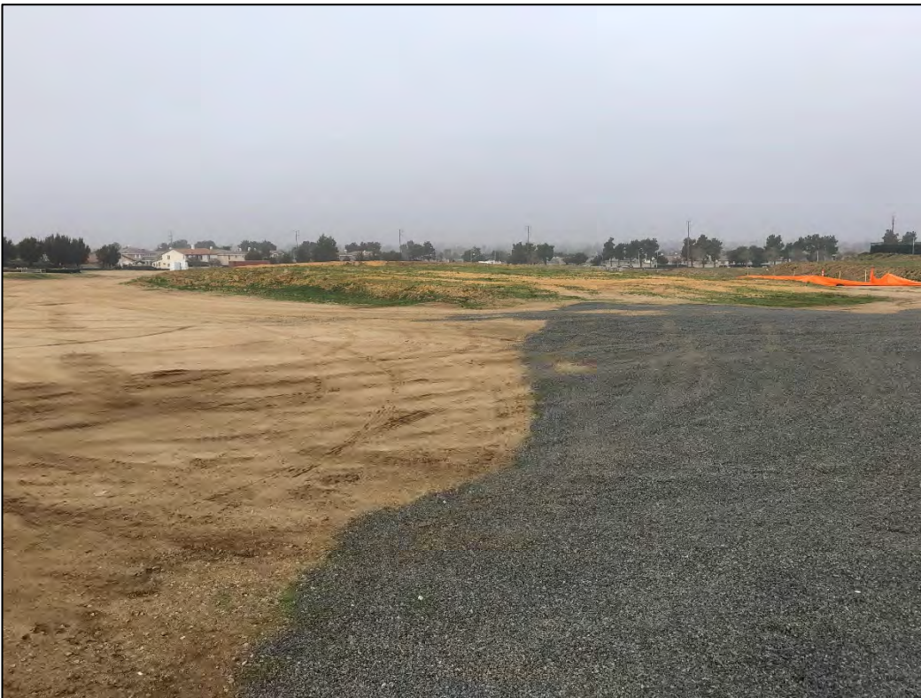
Looking north-east across the Project site.
