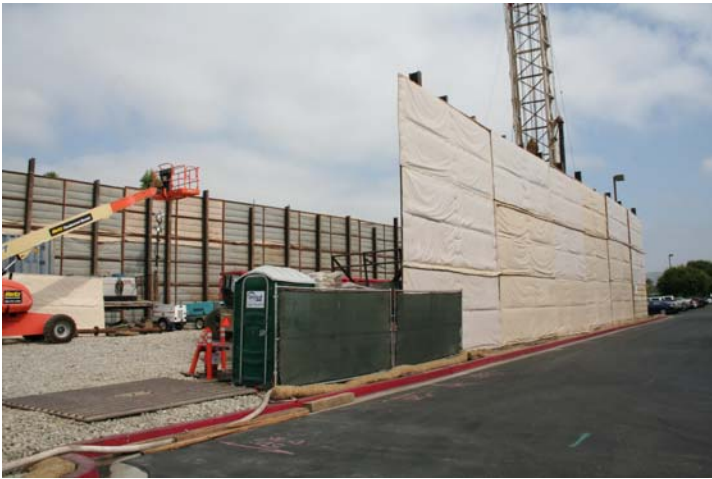
I-Beam & Acoustic Material 03
