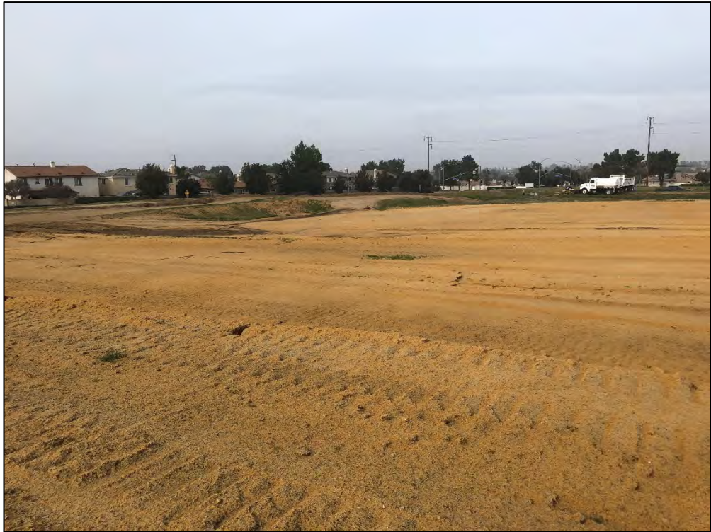
Looking north-west across the Project Site.
