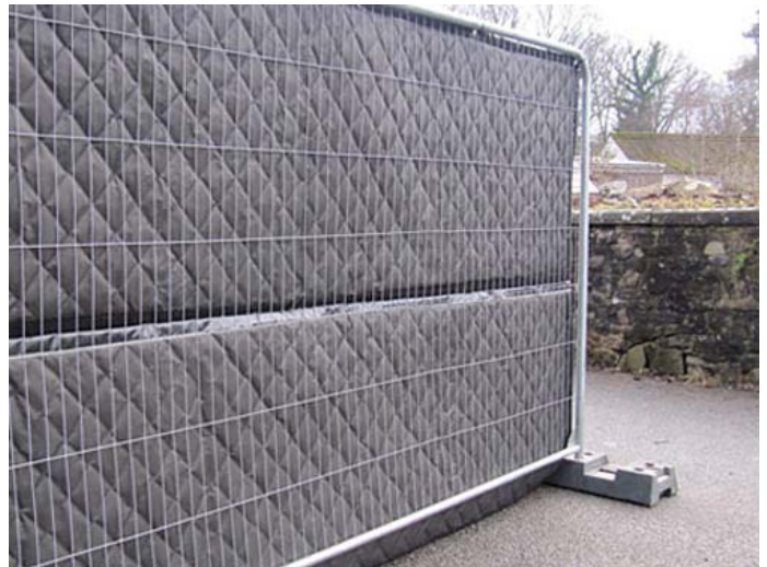
Temporary Fence & Acoustic Material 01
