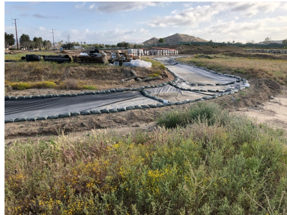
Figure 9: Photo of Drainage Channel Running From Northern Center Edge of Site to Southwestern Corner.
