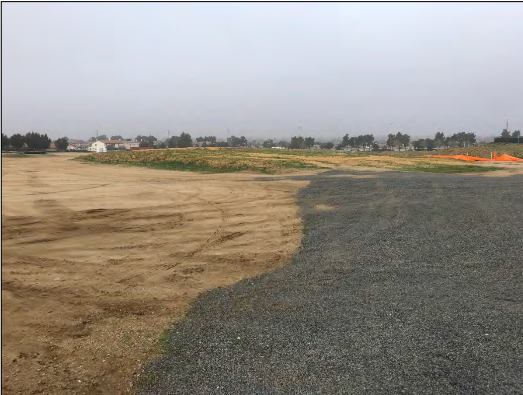
Looking north-east across the Project site.
