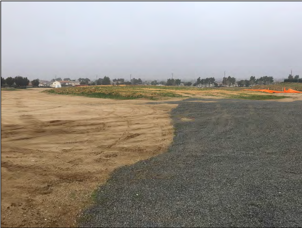
Looking north-east across the Project site.
