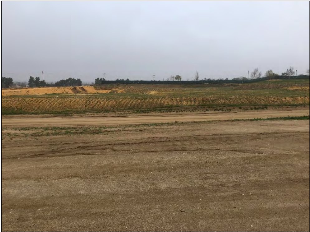
Looking east across the Project site at the previously graded development pads.
