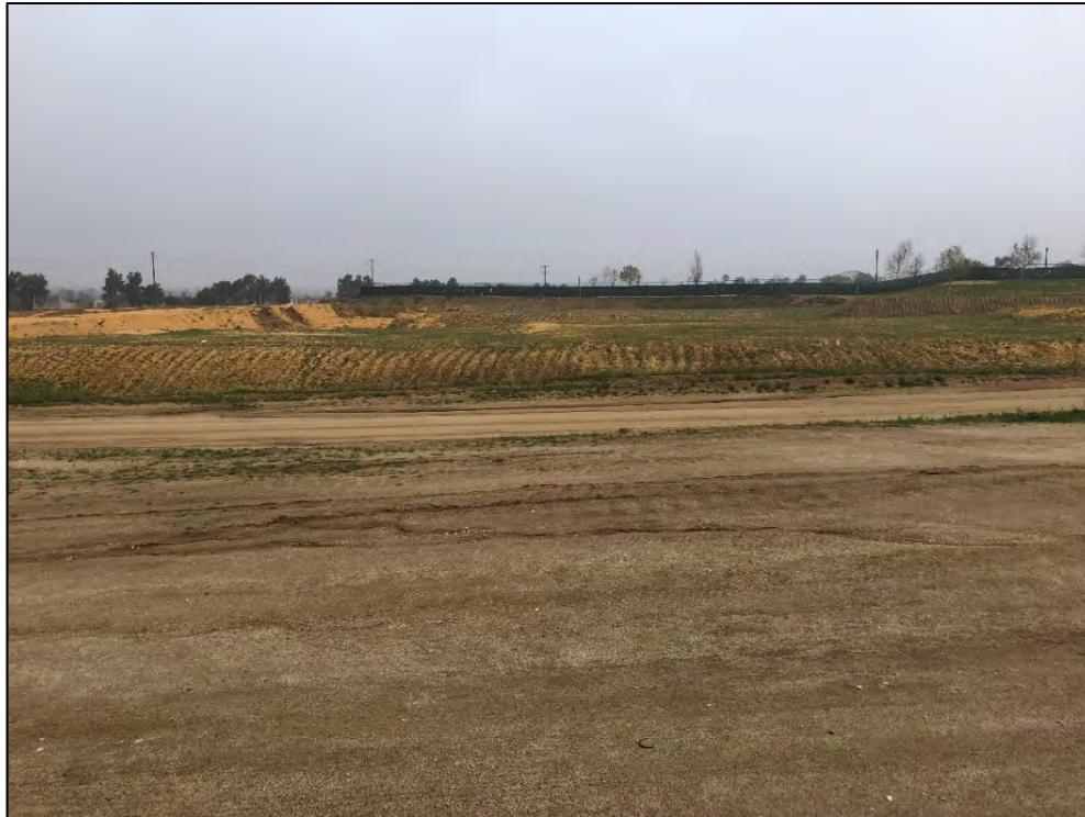
Looking east across the Project site at the previously graded development pads.
