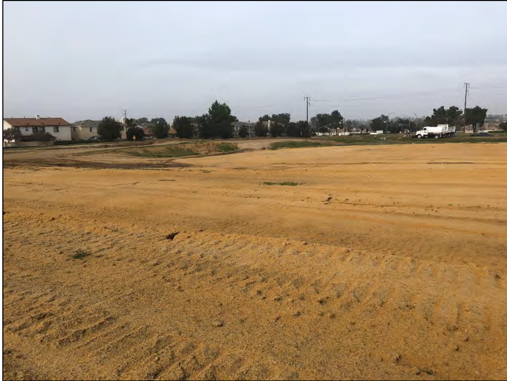
Looking north-west across the Project Site.
