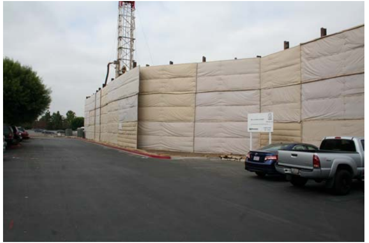
I-Beam & Acoustic Material 02
