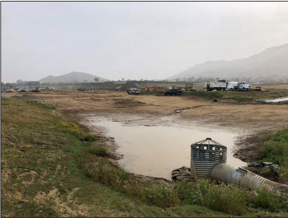
Retention Basin located on the northwestern most portion of the site to capture and retain the nuisance water and runoff.
