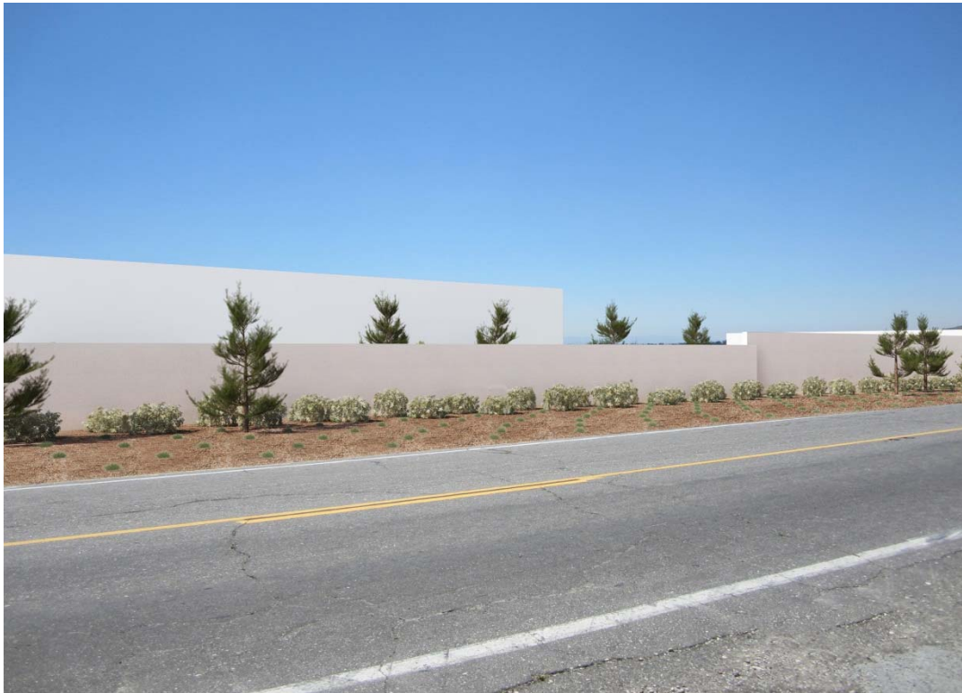
Gilman Springs Rd. View 5 at Installation
