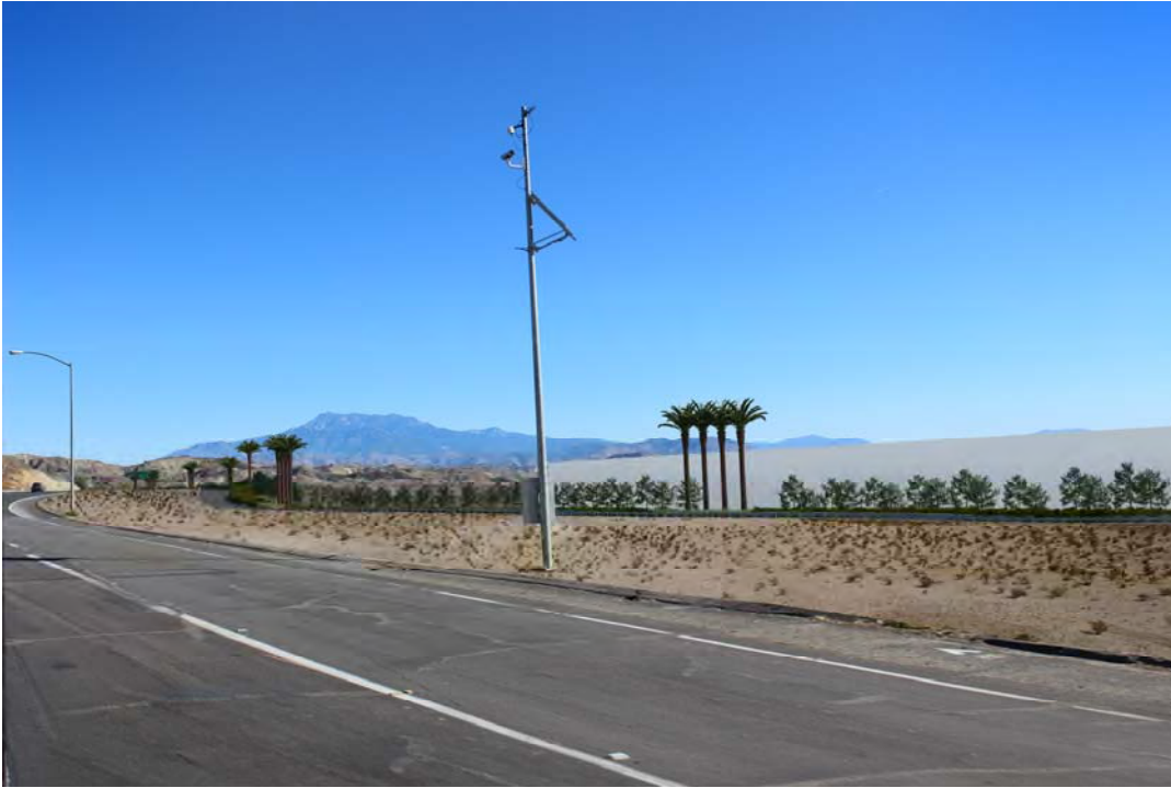
60 Freeway View 7 at Installation
