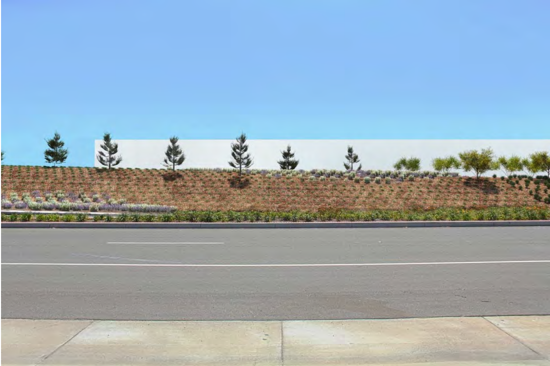
Redlands Blvd. View 1 at Installation
